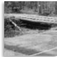
Pole bridges can be used for temporary crossings under certain conditions.
